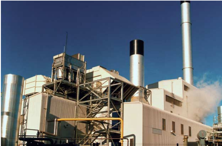
The CHP plant at British Sugar's Wissington Factory
