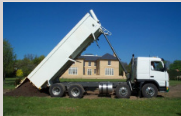
Topsoil being delivered and applied
