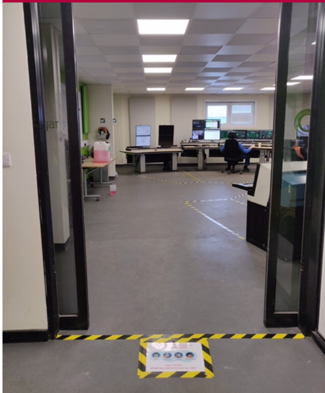
British Sugar control room segregation
