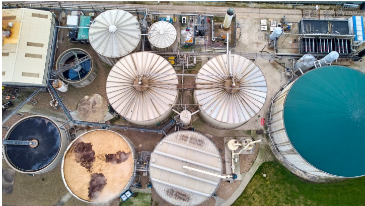
The anaerobic digestion facility at AB Mauri's yeast plant in Hull, UK
