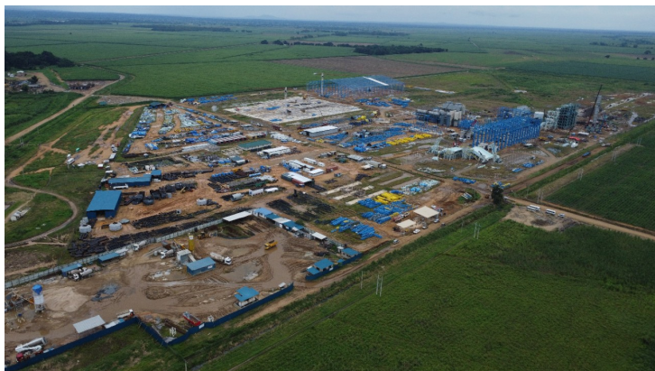
The K4 sugar factory and warehouse under construction at Kilombero in Tanzania
