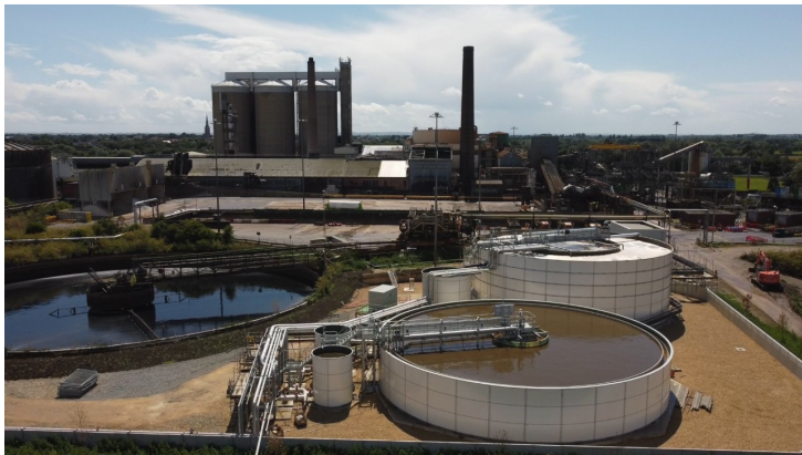
New water treatment facility, Newark, UK
