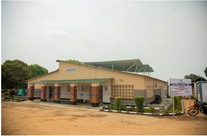
The Nakambala Urban Clinic, a health facility in Mazabuka, Zambia, that was refurbished with funding by Zambia Sugar in 2023
